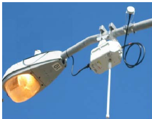
Figure 8-3 1500 Series Mesh AP Installation
